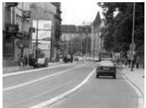
Fig. 5. ul. Grzegórzecka in Cracow. (a) prior to retrofit in 1999; and (b) following kerb separation of tram tracks/bus lane in 2000
